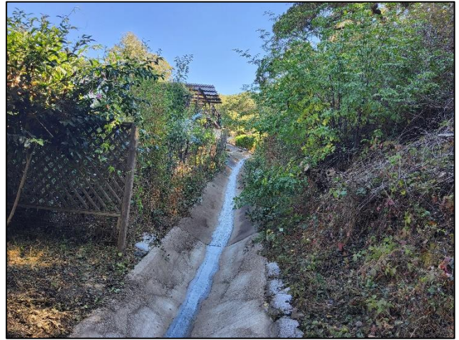
Photo 0927. Enhanced drainage in project area, view to NE
